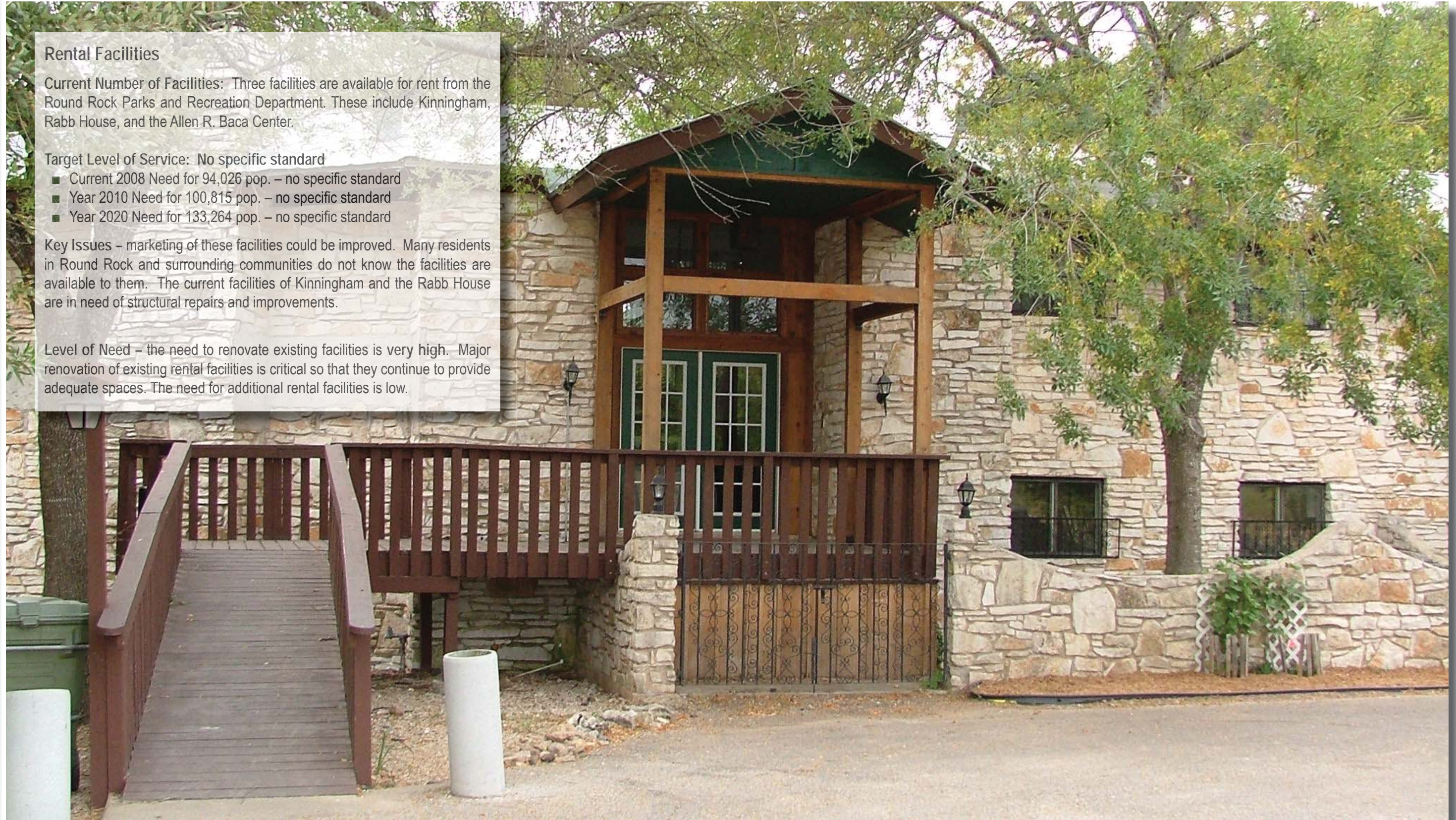
Rabb House, in need of significant renovation.
