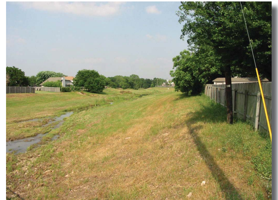
Incorrect Model - Unattractive drainage corridor in the city that could have served as a trail and park corridor. Lots backing up to the corridor create a "no-man's land" that serves only to carry stormwater.
