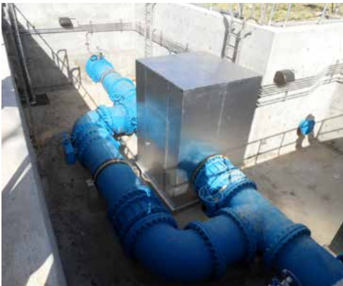
Control Valve vault on Treated Water Segment 3 Project.
