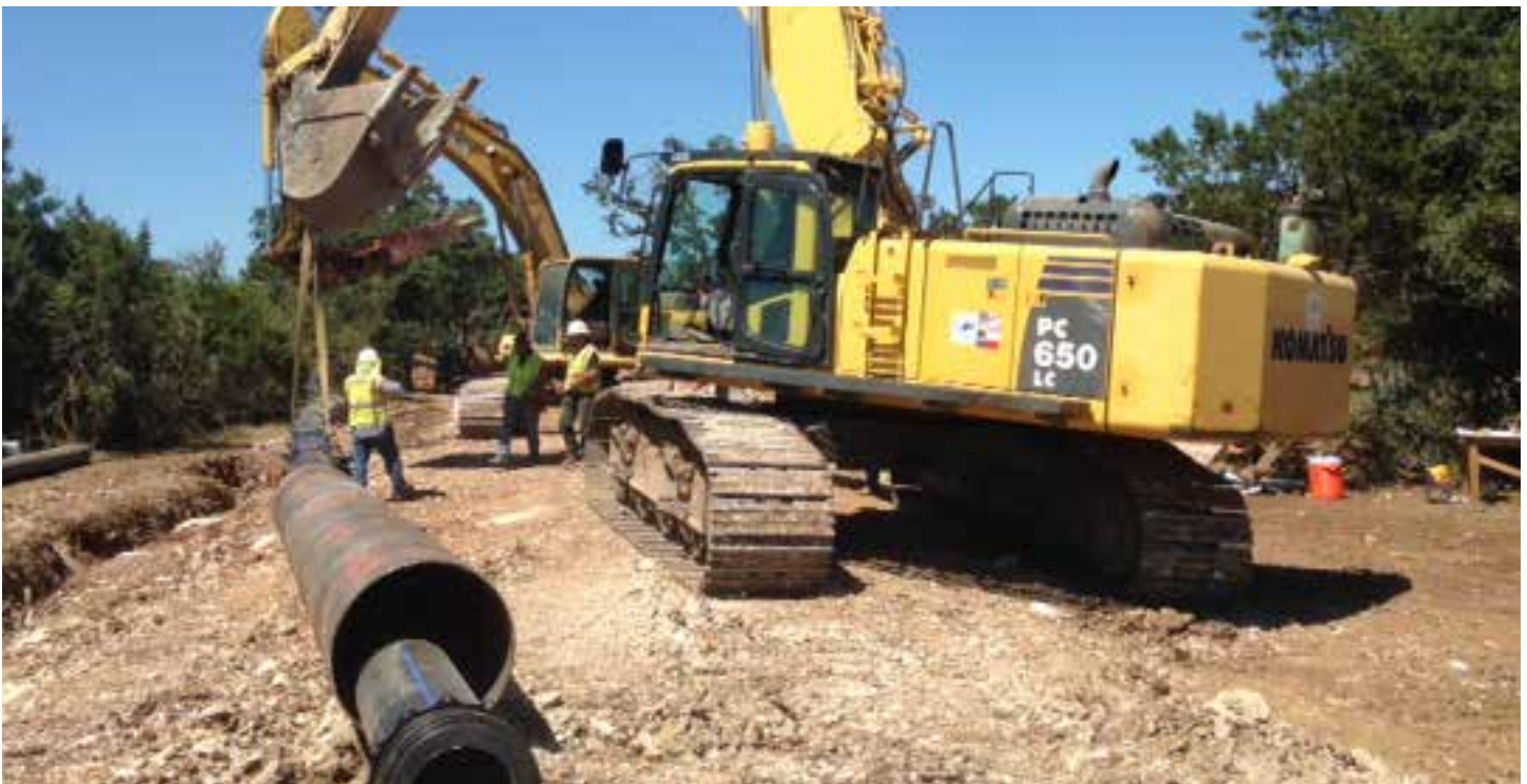
16" fused HDPE pipe with steel casing on the Arterial H 16" Waterline Project.
