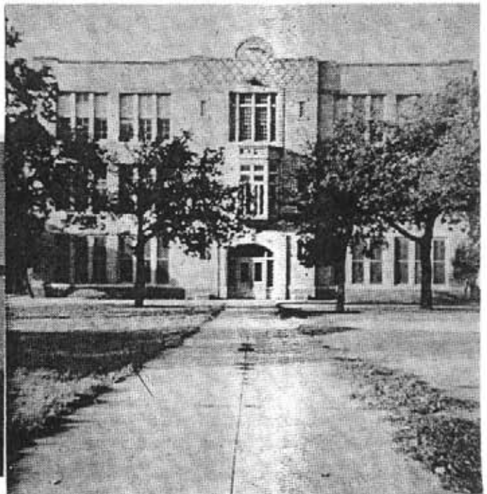
THREE-STORY PUBLIC SCHOOL BUILDING 1914-1959
