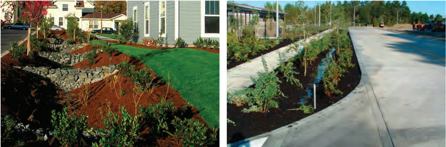
Street-edge bio-swales for the collection of rain water.
