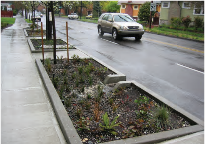
Rain garden with pebbles and plants creates permeable surface, absorbing and filtering rain water from street during storm.
