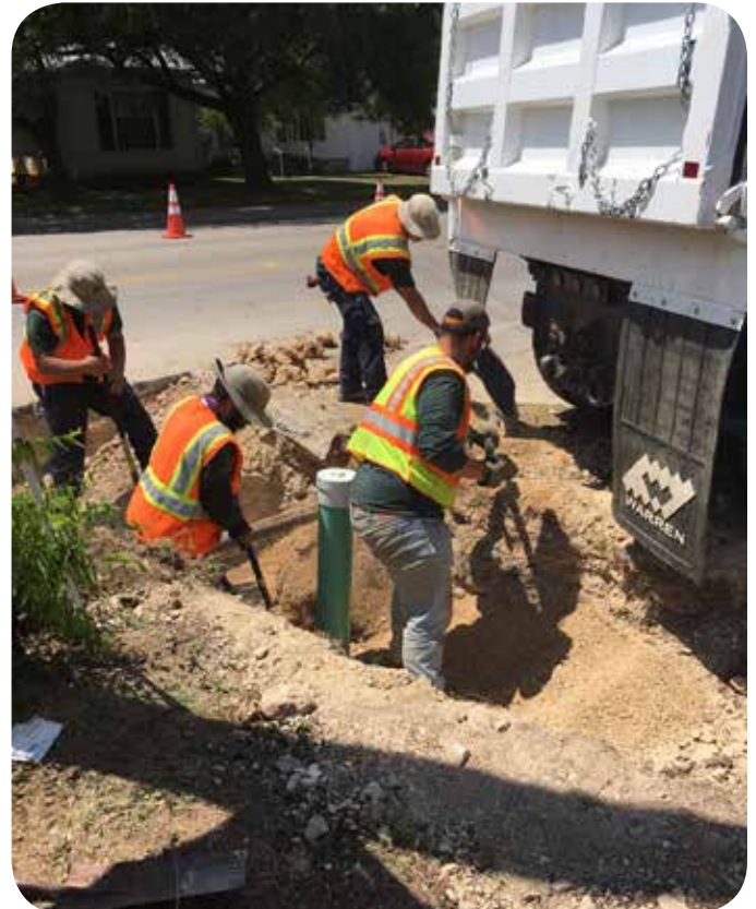
Wastewater Tap & Tie-in that the crew did to tie in a customer to an existing wastewater line. This occurred on North Georgetown Street
