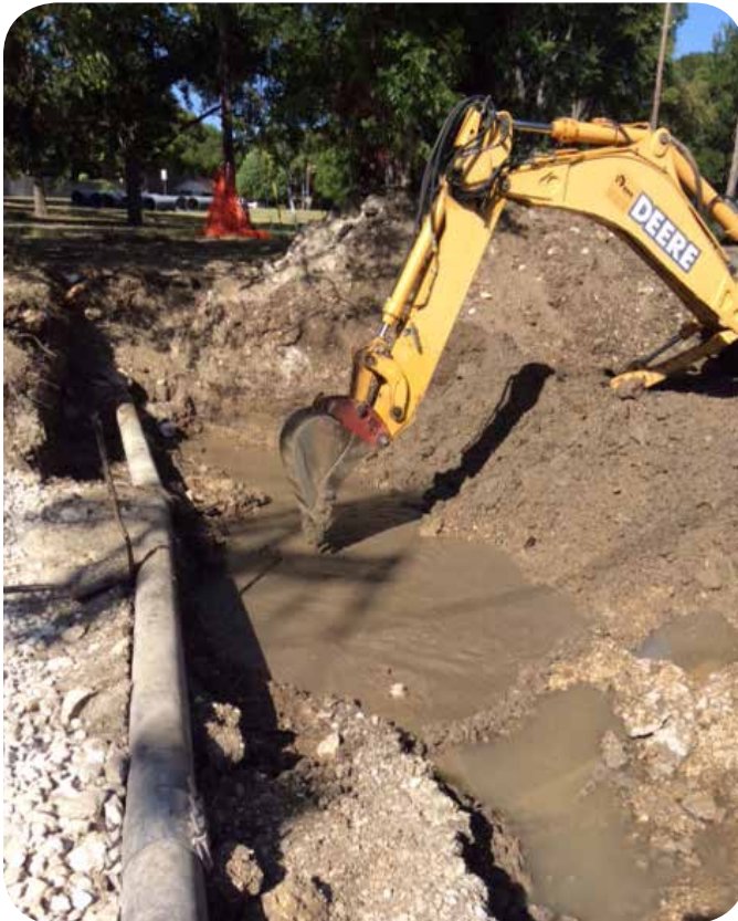
Moving of a Waterline in order to redo/move a bridge at Laker Creek
