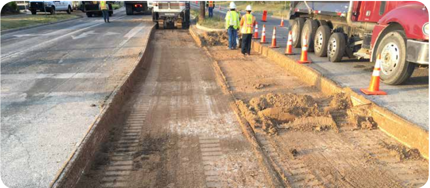
Milling The NB LTL Deep Wood #6. Photo taken on July 2017
