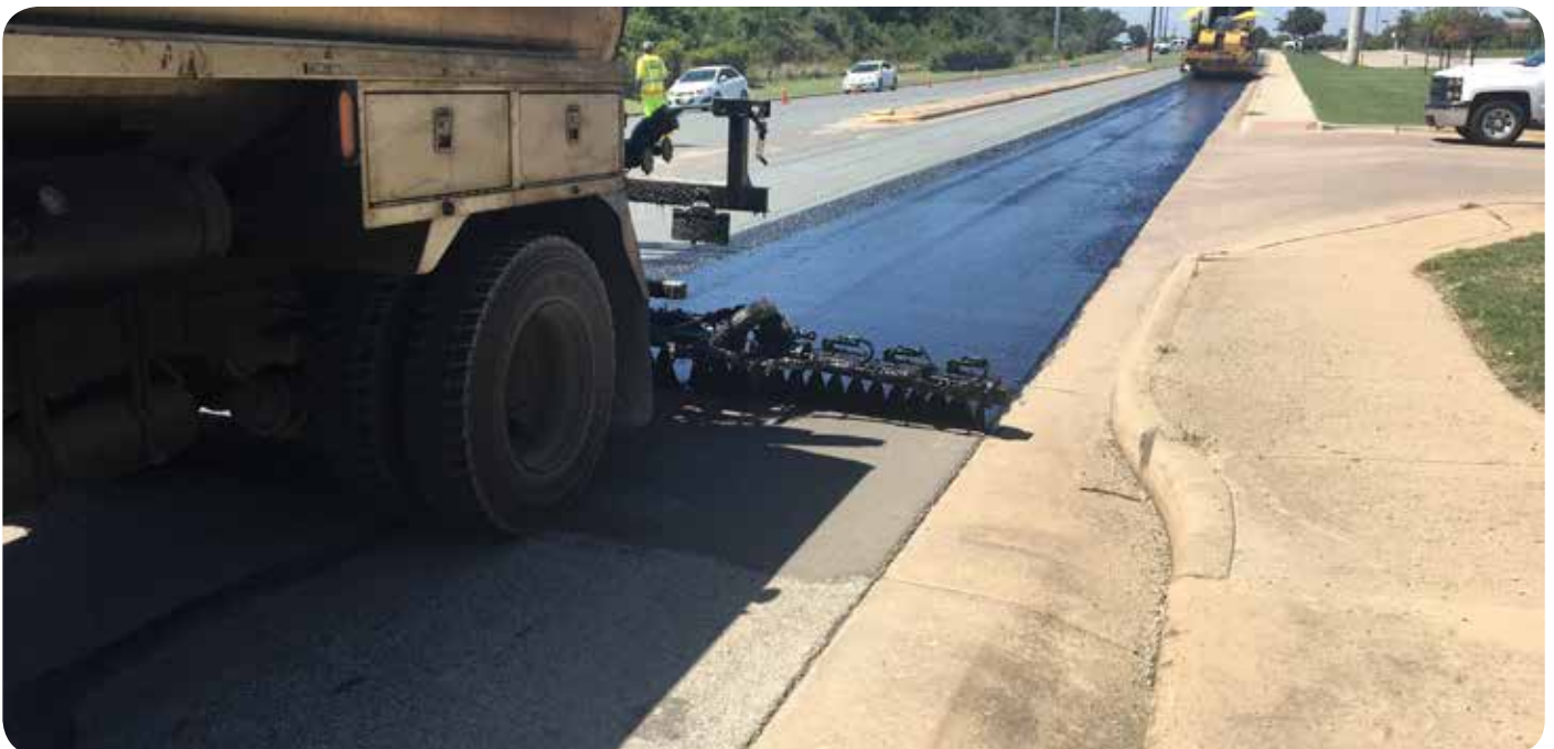
Transportation crews repaving Deep Wood Drive
