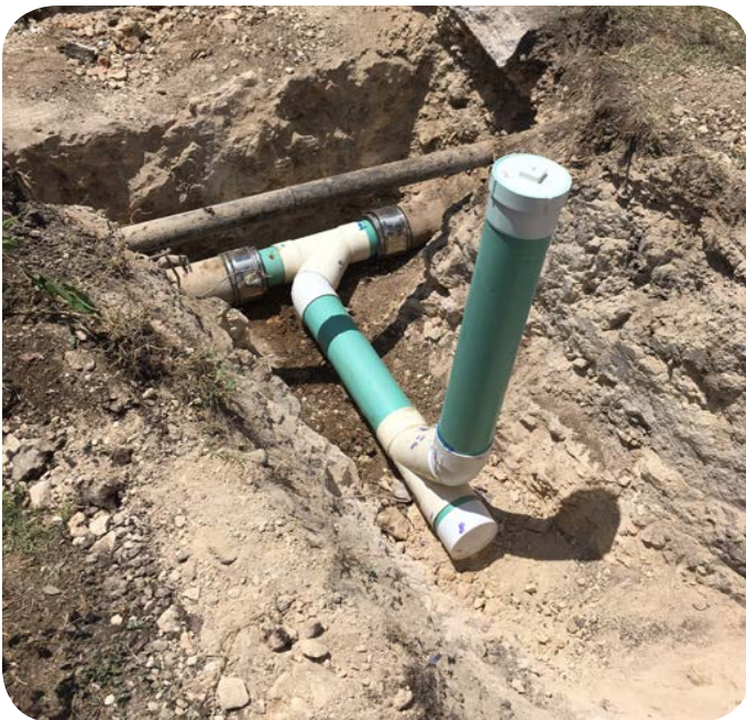
Wastewater Tap & Tie-in that the crew did to tie in a customer to an existing wastewater line. This occurred on North Georgetown Street.
