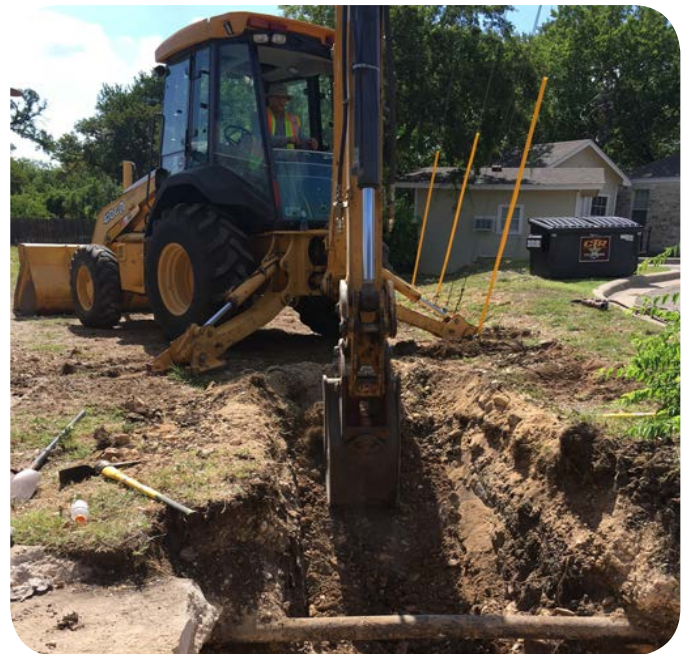
Wastewater Tap & Tie-in that the crew did to tie in a customer to an existing wastewater line. This occurred on North Georgetown Street.
