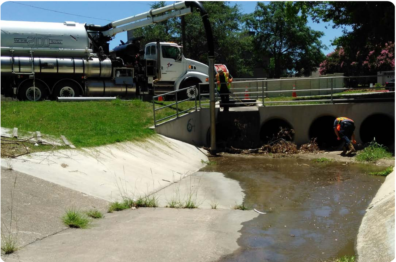
Drainage crews cleaning up drainage ditch
