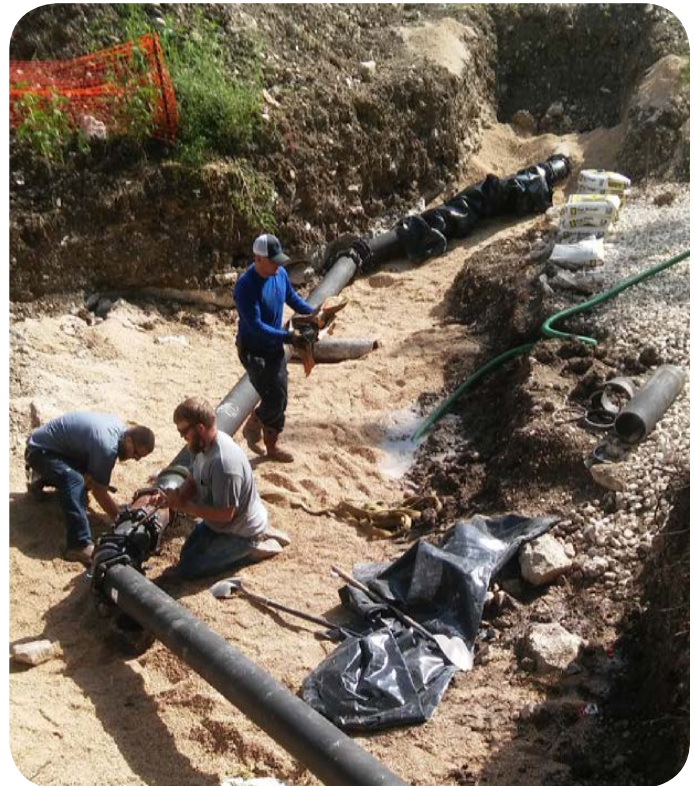
Waterline Maintenance moved a water line as Transportation had to redo/move a bridge that washed out in Lake Creek park.
