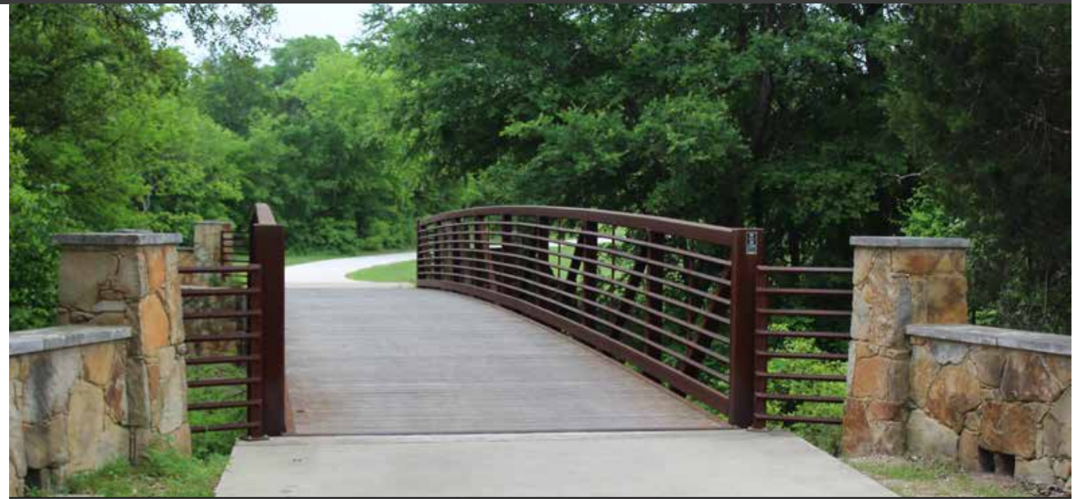
Foot Bridge - Brushy Creek Regional Trail
