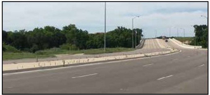
Existing section of Kenney Fort Boulevard Phase 1.
