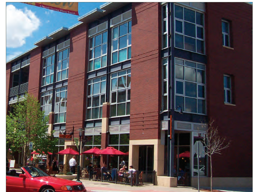
Large windows with minimal glazing face primary street with secondary entrance and smaller windows on secondary street.
