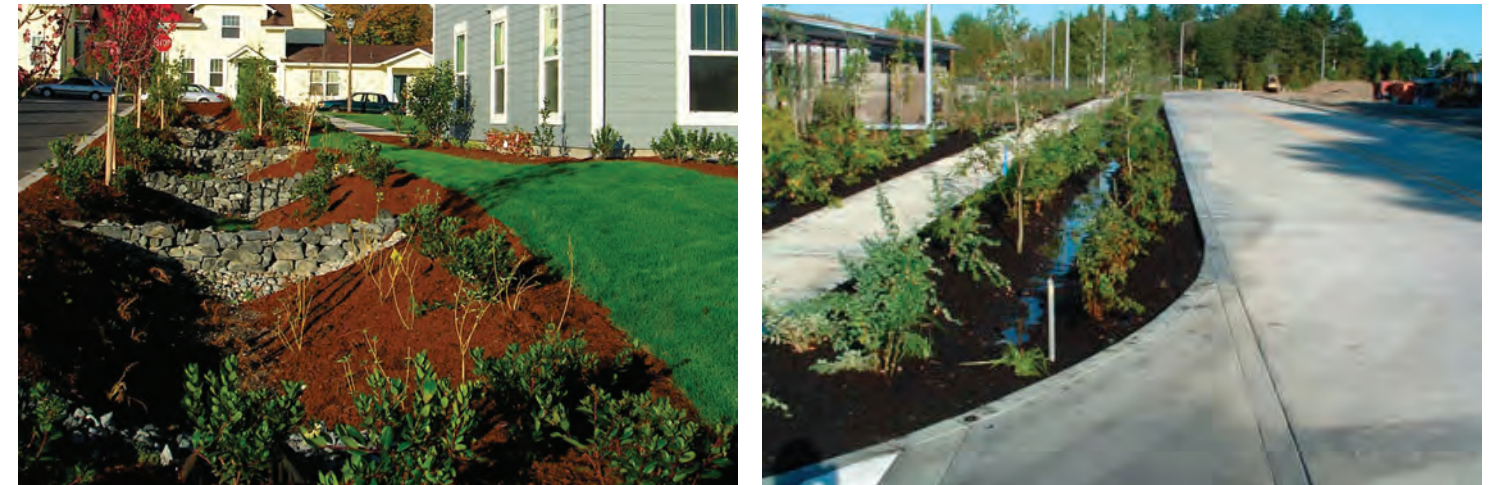
Street-edge bio-swales for the collection of rain water.
