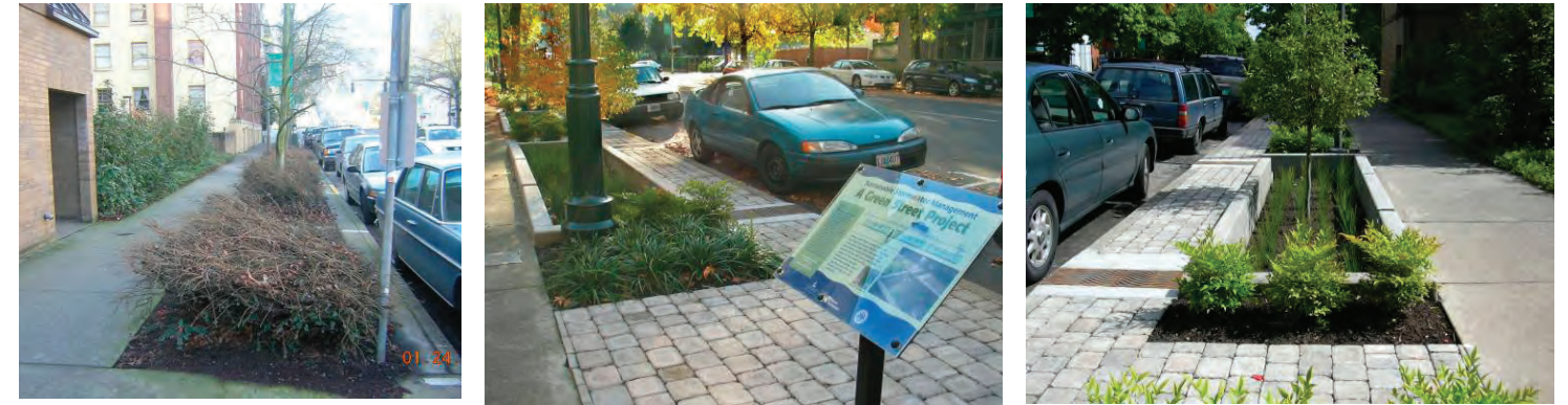
Portland "green street" before and after with rain garden, grate, and permeable bricks to collect and divert stormwater.
