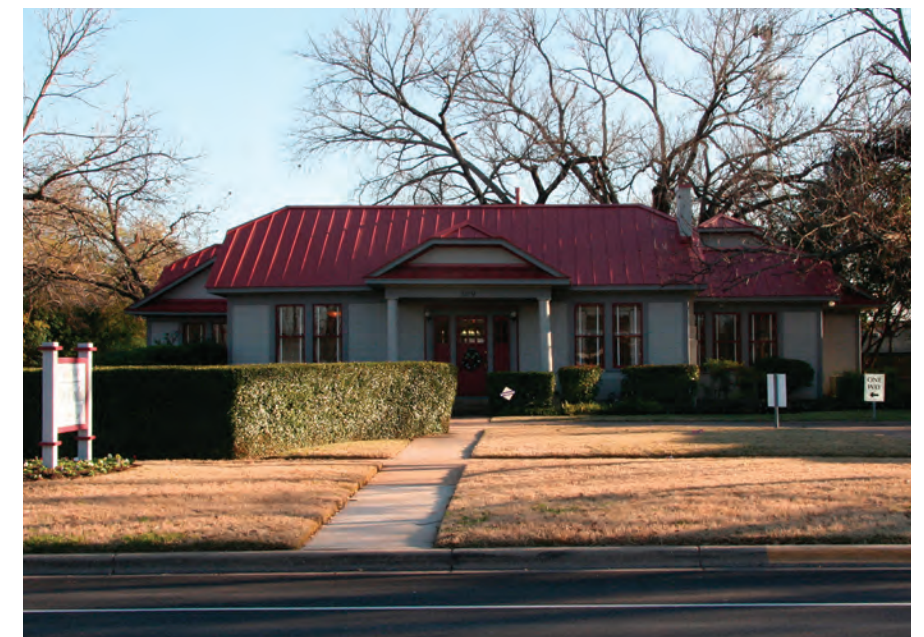
Adaptively-reused building at 309 E. Main Street.
