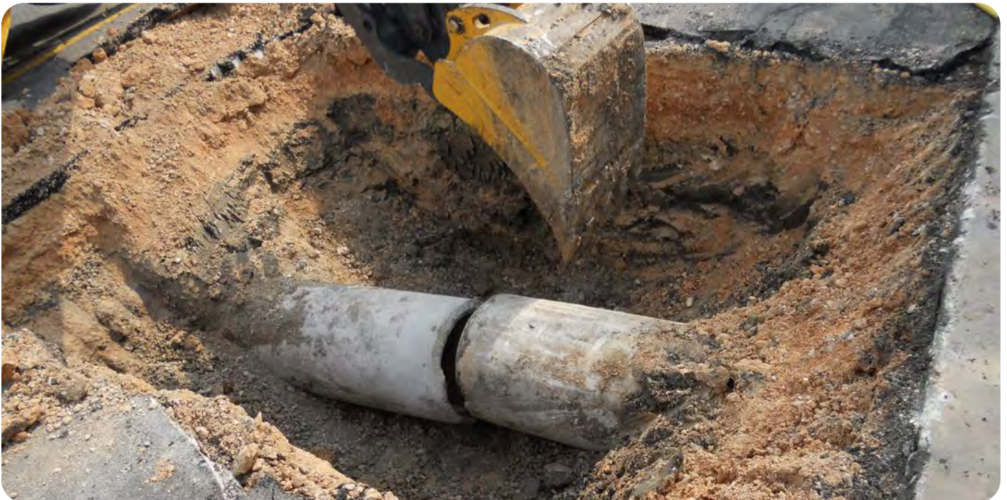
Drainage Pipe Repair
