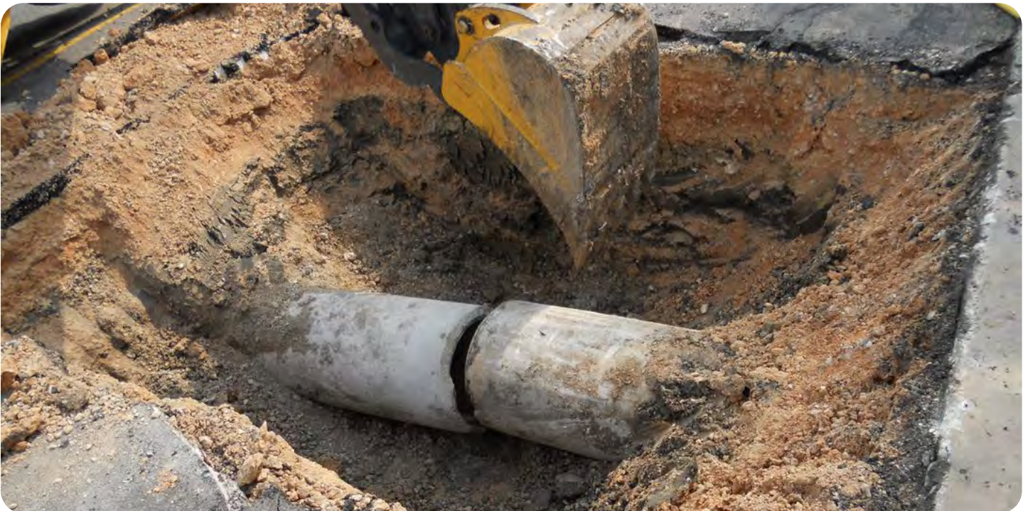
Drainage Pipe Repair
