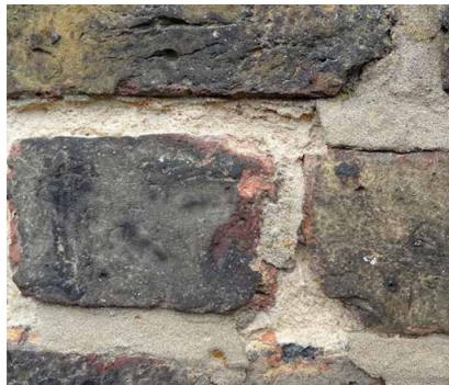
Crumbling cement layered over historic lime mortar. Photo from Historic England.
