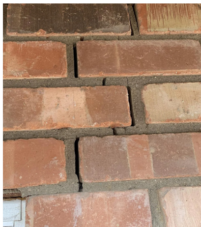
Broken bond between brick and mortar. Photo from Reddit.
