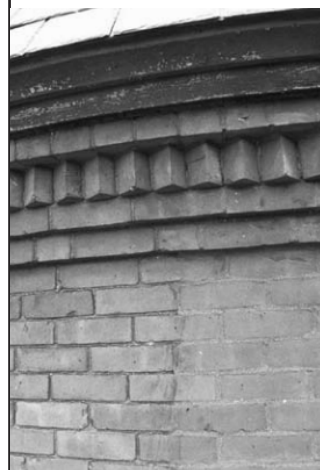
Poorly matched tooling depth. Photo from Sanders & Magness, 2007.
