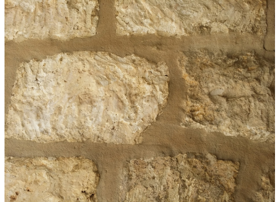
Successful repointing of a historic structure at Stagecoach Inn.
