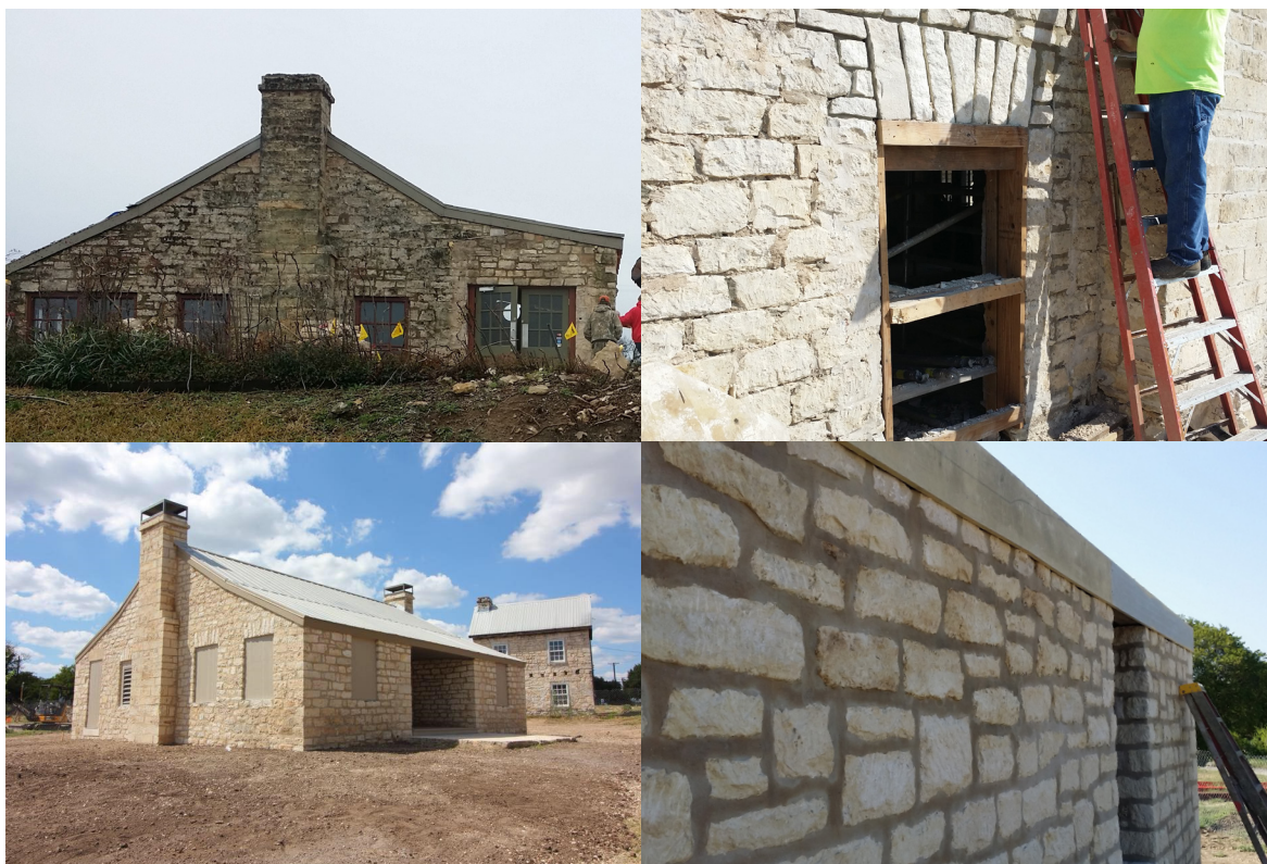
Clockwise, from upper left: before mortar repair and cleaning; joint preparation; after filling and tooling; finished building.
