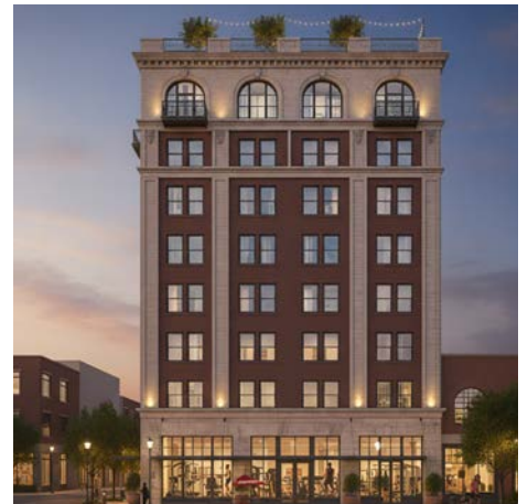
Gym at street level with offices above
