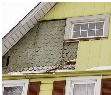
Synthetic siding removed to reveal original wood shingles
