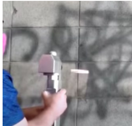
Removing spray paint from a stone wall using laser ablation
