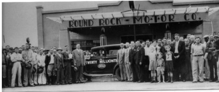
In 1930 the Round Rock Motor Co. was at 216 E. Main Street. The brick building was coated with stucco after a fire and given a more modern appearance. The building housed the city library in the 1960s.
