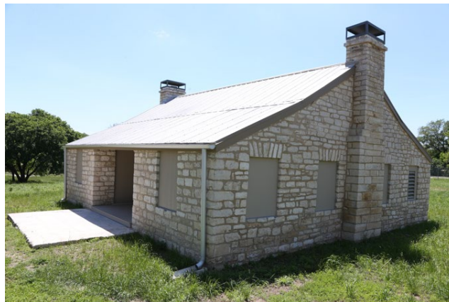
The historic Stagecoach Inn was mothballed until a rehabilitation plan was finalized
