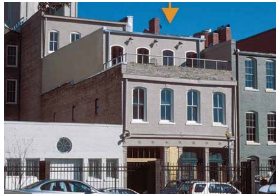
Rooftop addition in a commercial building.
