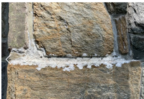
Efflorescence in masonry
