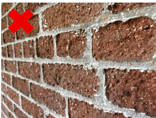
Brick damaged by aggressive pressure washing
