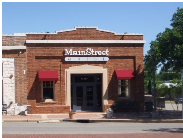
The Farmers State Bank building (built 1920) was built with small windows for security. The railroad and the development of local building supply businesses allowed brick and other manufactured materials to be more commonly used.
