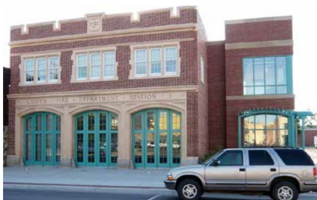
Addition to the historic building via an offset brick hyphen. The roof form, materials, and color are compatible, while the fenestration pattern is differentiated.
