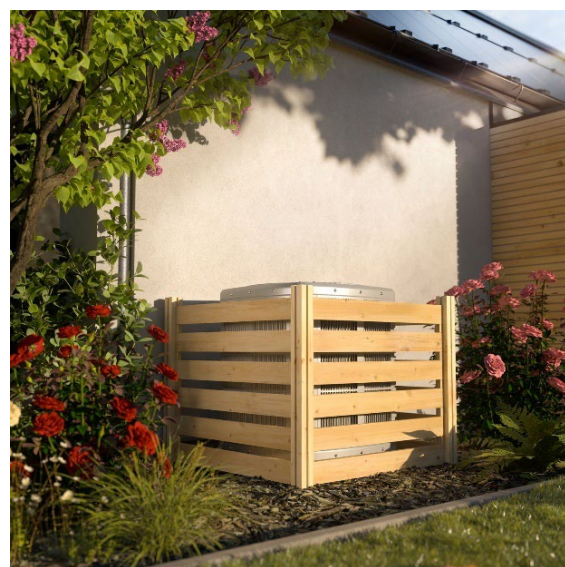
Mechanical equipment screened from public view
