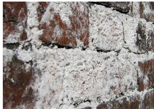
Efflorescence in masonry
