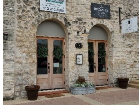
Example of a building that originally had paired doors which were replaced with single doors in the 1960s. Double doors similar to the original were restored in 2017.
