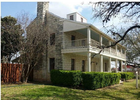
The Captain Nelson Merrell House (1871, National Register and City Landmark) was built for comfort in hot weather, with 18-inch-thick limestone walls and a full-length gallery on the south side. A valve on the gutters allowed rainwater to be directed into the cistern.
