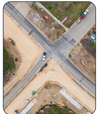
Chisholm Trail Widening
