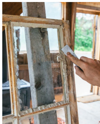
Top: Double-hung window components Bottom: Applying new glazing putty to wood windows
