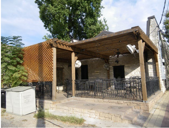
Covered patio with metal railing attached to the building
