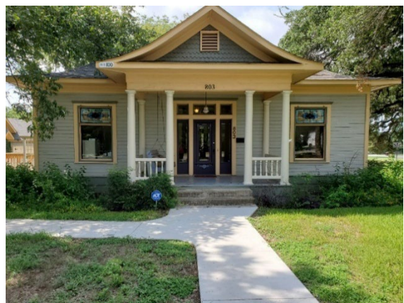
Typical Railroad era house on E Liberty with wood siding, sloped roof and front porch
