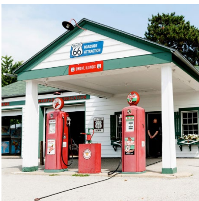
Vehicle canopies are key façade features of some commercial buildings
