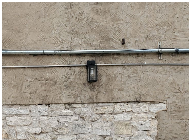
This wall received a scratch coat of stucco a century ago but never received a finish coat. It is best left in its historic condition and repaired as needed
