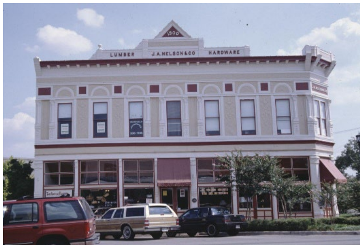
The Nelson Hardware Building (built 1900) used a storefront facade system from the Mesker Brothers of St. Louis to combine two existing limestone buildings that had been damaged by fire. The storefront system included wood-framed doors and windows as well as the pressed tin and cast-iron components.
