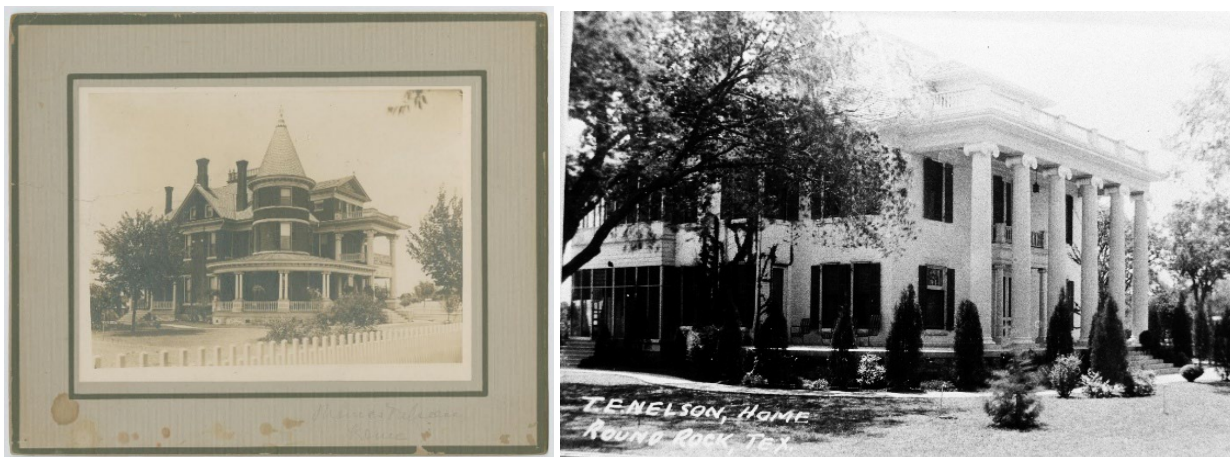
The Nelson-Crier House (a.k.a. Woodbine Mansion), completed in 1900, was originally built in a Queen Anne style with a porch that wrapped around the base of a three-story turret (Left). In 1931 The owners restyled the façade to Classical Revival by removing the turret and installing a six-column porch
