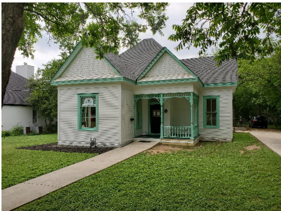
This Queen Anne style cottage on E. Main Street (ca. 1900, City Landmark) was home to the Black and Engstrand families, early retailers.
