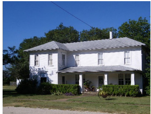
The William J. Walsh House (1905, City Landmark) was originally a Folk Victorian. It is not known whether it was remodeled as a Craftsman in response to damage or for the then-owner's preference.
