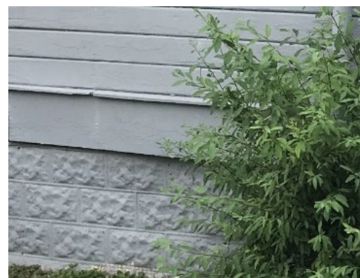
Pressed metal skirting with historic rough stone pattern
