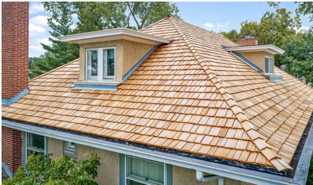
Cedar Shake Roof
