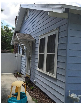
Wood siding (right) restored after it had been covered with vinyl siding (left)
