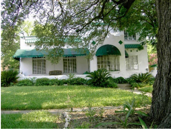
The Walsh House once had large fabric awnings on the south side.
