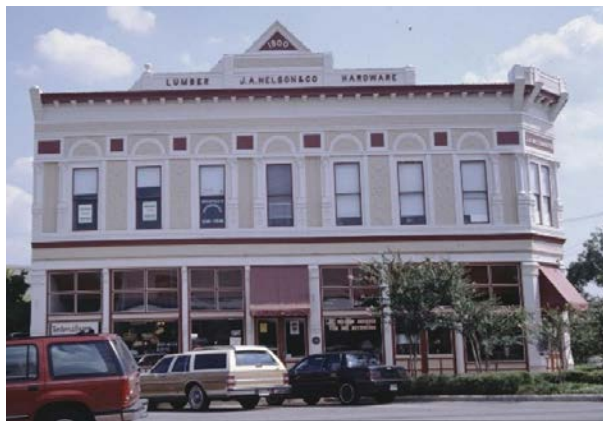
The Nelson Hardware Building (built 1900) used a storefront facade system from the Mesker Brothers of St. Louis to combine two existing limestone buildings that had been damaged by fire. The storefront system included wood-framed doors and windows as well as the pressed tin and cast-iron components.
