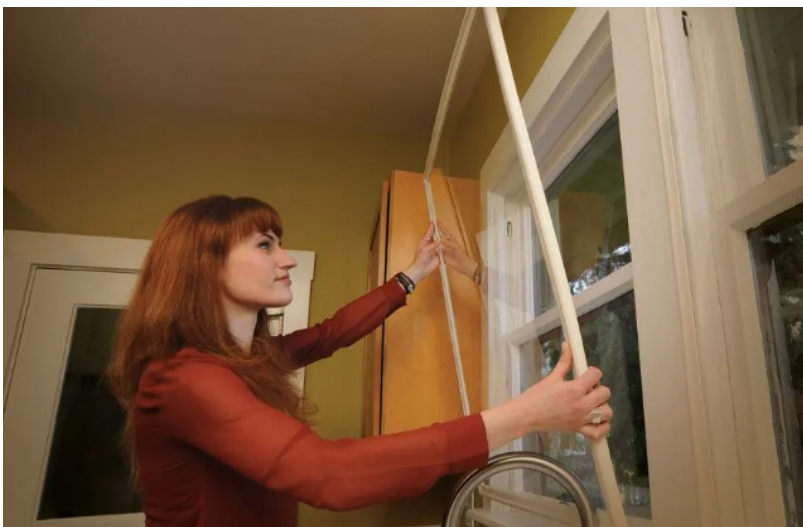
Interior storm windows offer the benefits of traditional storm windows without affecting the exterior appearance and may easily be removed when occupants wish to open a window.
