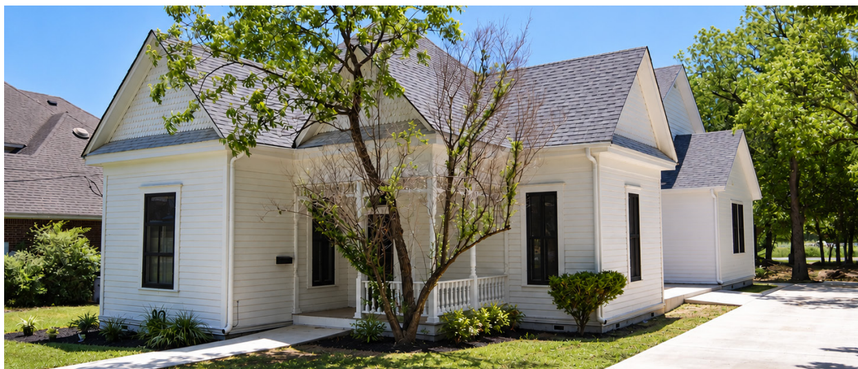
This 2018 rear addition attached with the simple connector complements the original ca. 1899 house with compatible form and massing. The original structure's form also remains intact.
