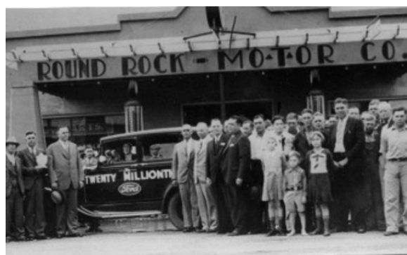
In 1930, the Round Rock Motor Co. was at 216 E. Main Street. The brick building was coated with stucco after a fire and given a more modern appearance. The building housed the city library in the 1960s.
