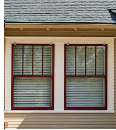
Craftsman style, double-hung windows often had a multiple-lite upper sash with a single-lite lower sash
