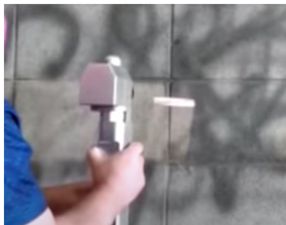
Removing spray paint from a stone wall using laser ablation
