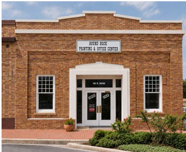
Offices and banks had little or no need for display, and windows were sized to provide light to the interior.
