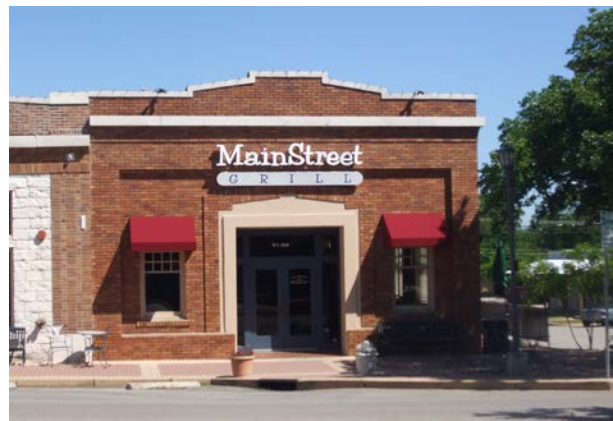
The Farmers State Bank building (built 1920) was built with small windows for security. The railroad and the development of local building supply businesses allowed brick and other manufactured materials to be more commonly used.
