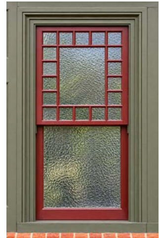
Victorian style, multi-pane double-hung window with privacy glass
