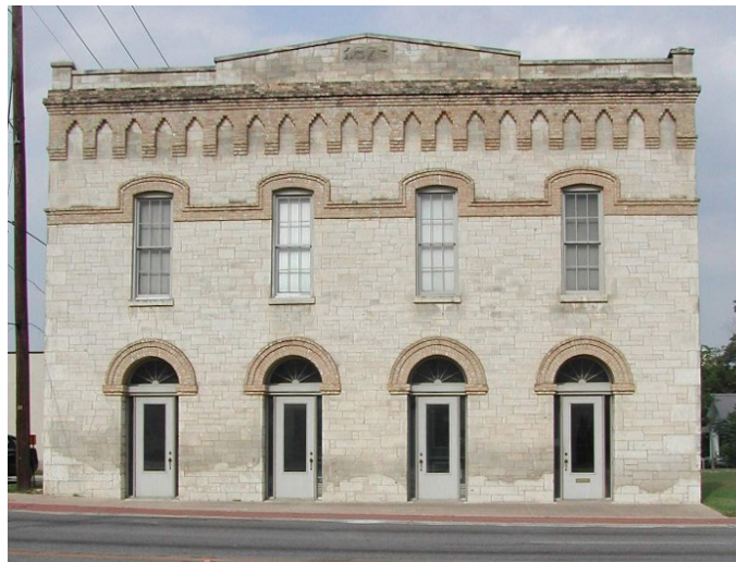
The Old Post Office/Masonic Lodge (built 1878)
