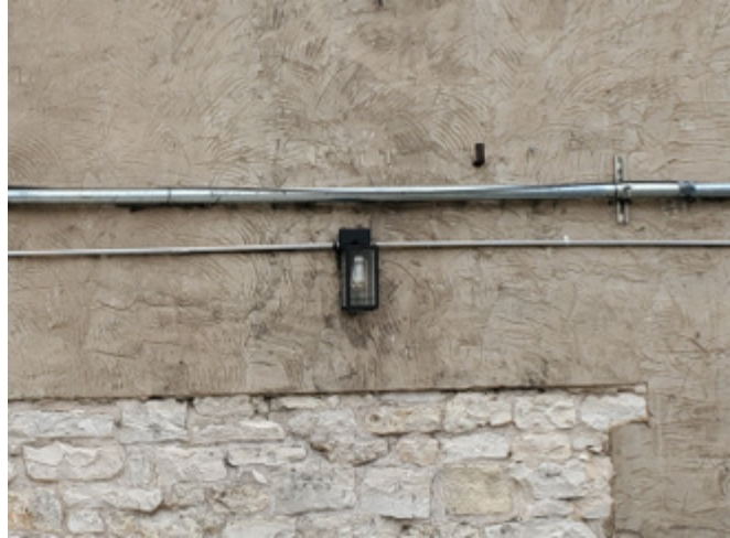
A century ago, this wall received a scratch coat of stucco but did not receive a finish coat. It is best left in its historic condition and repaired as needed.
