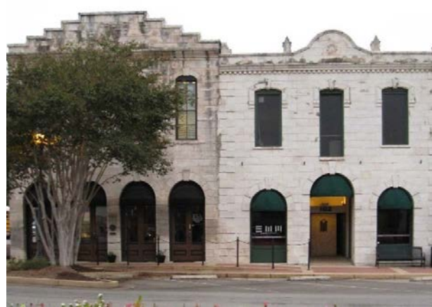
Later construction shows more refined stonework. The Old Broom Factory Building (built 1880, left) has smooth ashlar limestone. The Otto Reinke Building (built 1878, right) has a lime plaster finish scored to imitate carved stone. Both are in the Downtown Historic District, listed on the National Register of Historic Places.
