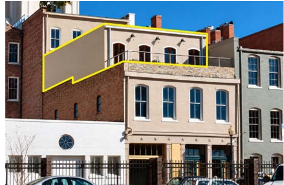
Rooftop addition on a commercial building
