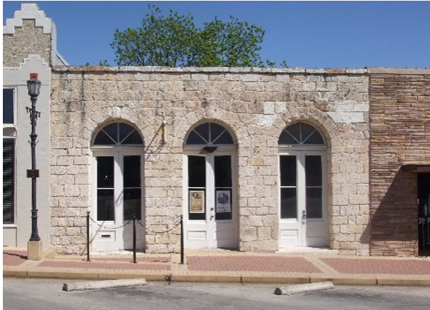
Early storefronts like the Round Rock Leader building (built 1881) had simple facades consisting of paired doors often with transoms. The design was adaptable to different businesses, providing sufficient air circulation and display space. The interior could be subdivided so that each tenant had their own entrance.
