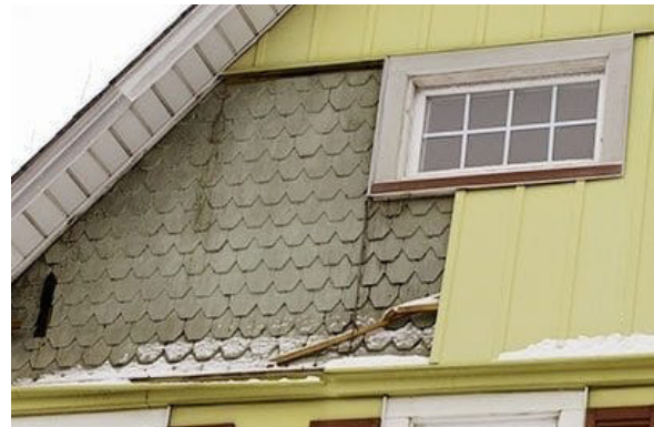
Remove synthetic siding to reveal original wood shingles
