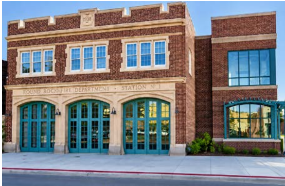
Right side addition to the historic building with offset and connector. The roof form, materials, and color are compatible, while the fenestration pattern is differentiated.
