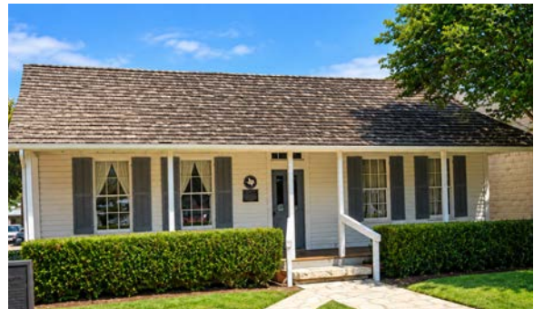
Most early homes in Round Rock originally had wood shake or shingle roofs.
