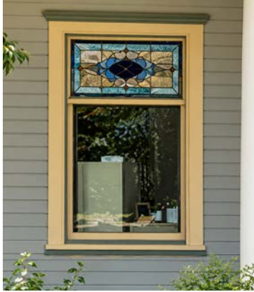
Victorian era fixed stained glass panel over single-lite operable window
