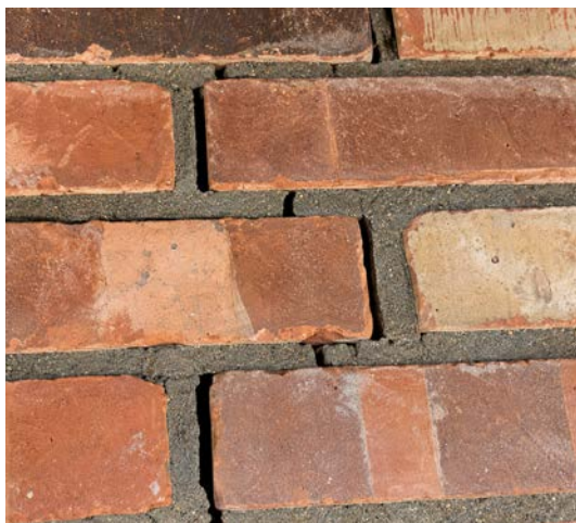
Examples of mortar joint failure
