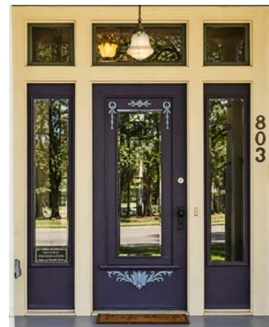
Front door with transoms and sidelights
