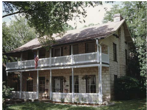
The Owen House, aka St Charles Hotel (built ca. 1870, National Register and City Landmark) was the residence of Dr. William M Owen, a prominent physician and businessman.
