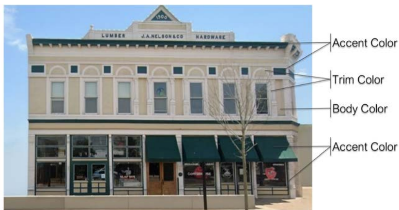
The Nelson Hardware Building (1900) uses a three-color scheme (beige walls, cream trim, green accents) to highlight the detail in the pressed-tin façade.
