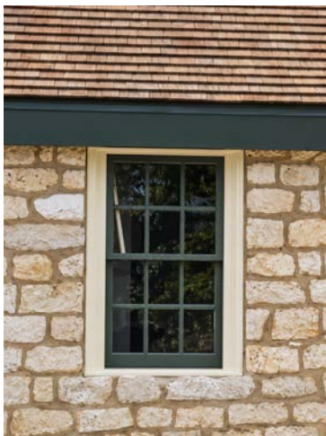
Simple six-over-six double hung window on a traditional, Pre-Railroad era house.
