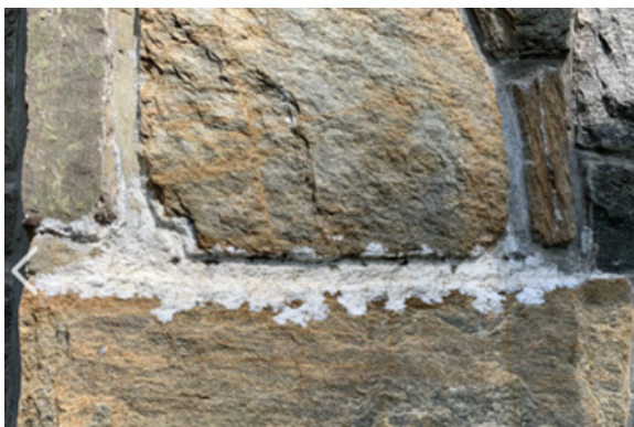
Efflorescence in masonry
