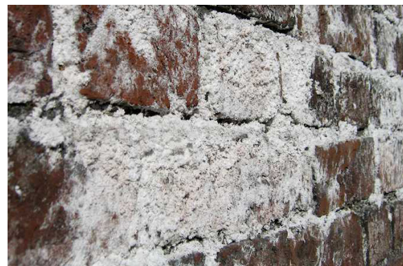
Efflorescence in masonry
