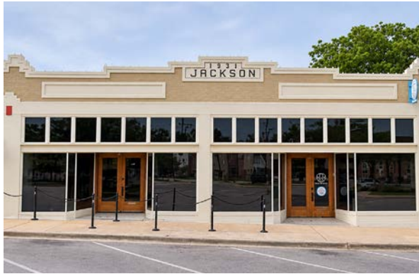
Storefronts feature large display windows. (Left) Transom windows above helped to direct light toward the back of the building, as the side walls were shared with adjacent buildings.
