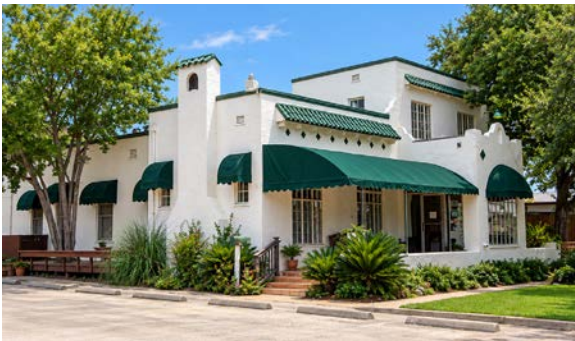
Some house styles are characterized by specific roofing materials, such as the glazed tile pent roof, chimney cap, and coping on this Spanish Revival home.
