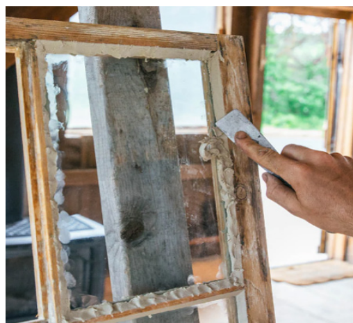
Applying new glazing putty to wood windows
