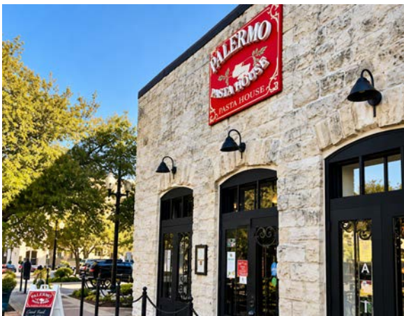
Shielded gooseneck lights used on downtown historic commercial building
