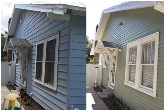
Wood siding (Right) restored after it had been covered with vinyl siding (Left)
