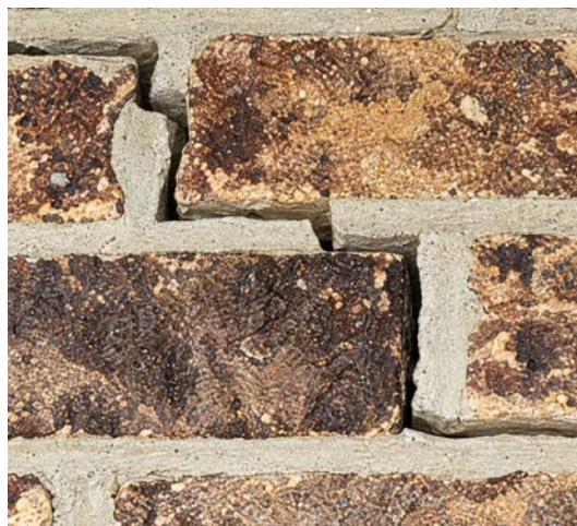
Examples of mortar joint failure
