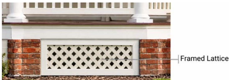
Masonry with framed lattice panels
