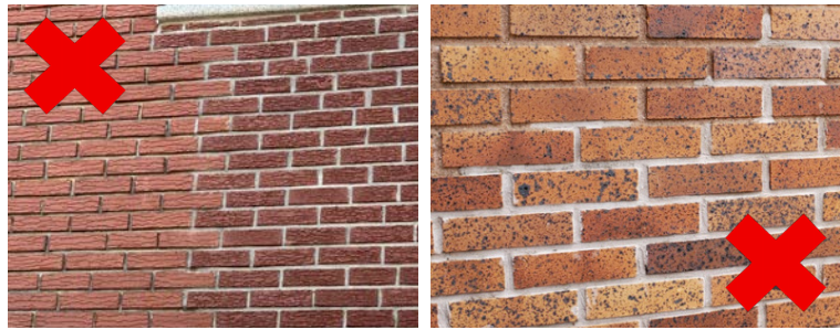
Poor matches for mortar color and tooling
