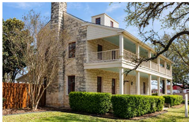
The Captain Nelson Merrell House (National Register and City Landmark) was built ca. 1871 for comfort in hot weather, with 18-inch-thick limestone walls and a full-length gallery on the south side. A valve on the gutters allowed rainwater to be directed into the cistern.
